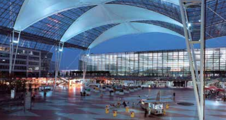
München Airport Center (MAC)
