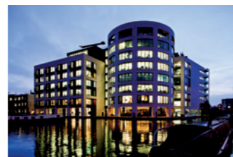
Barrackhorse Basin © John Sturrock
