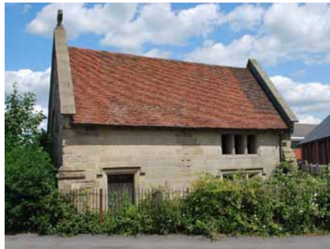
Restored chapel of the former leper hospital Martin Haslett © RGS-IBG Discovering Britain
